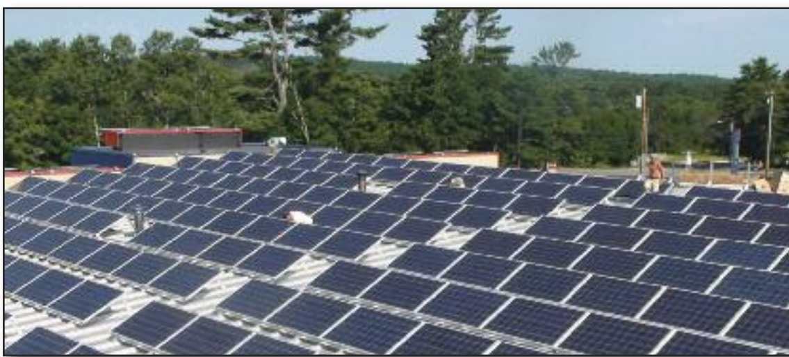
LMT Metal fabrication developed framing system for solar panel installations.
